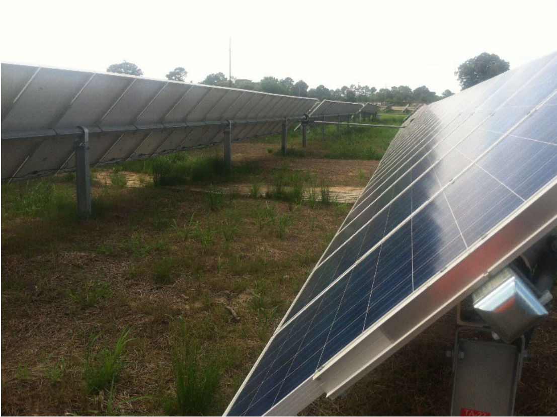
Wire management is completed.
