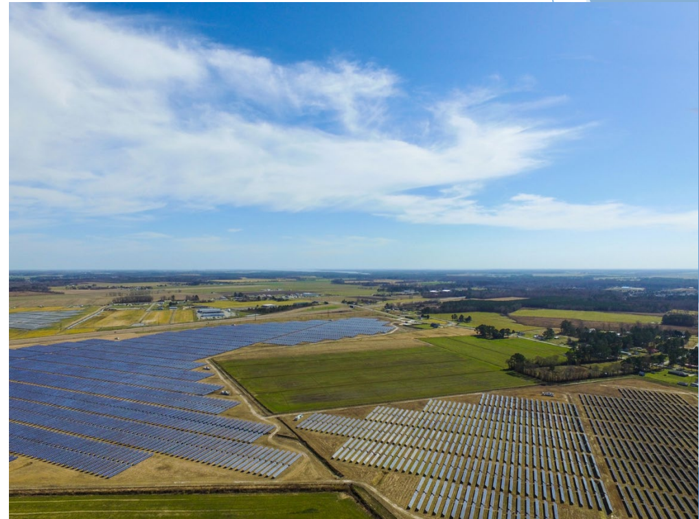
System is completed.
