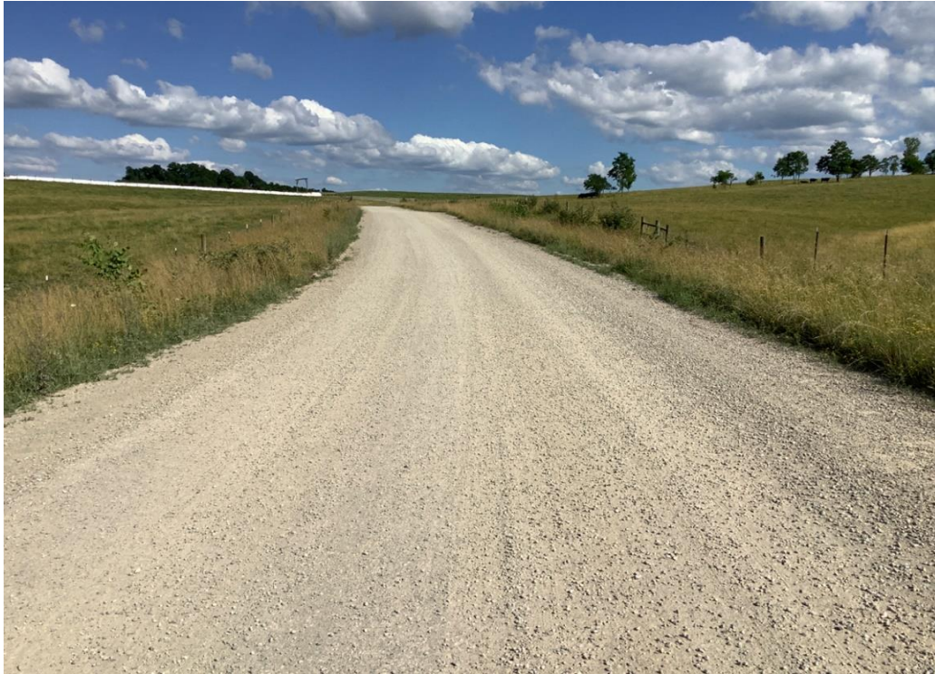
PHOTO 31: Typical aggregate pavement section of Luther Jones Road, looking east.
