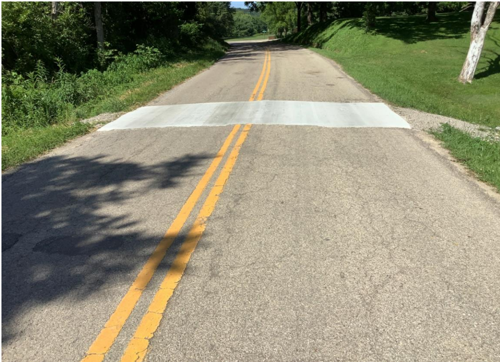
PHOTO 24: Pavement repair over culvert on Keystone Furnace Road, looking north.
