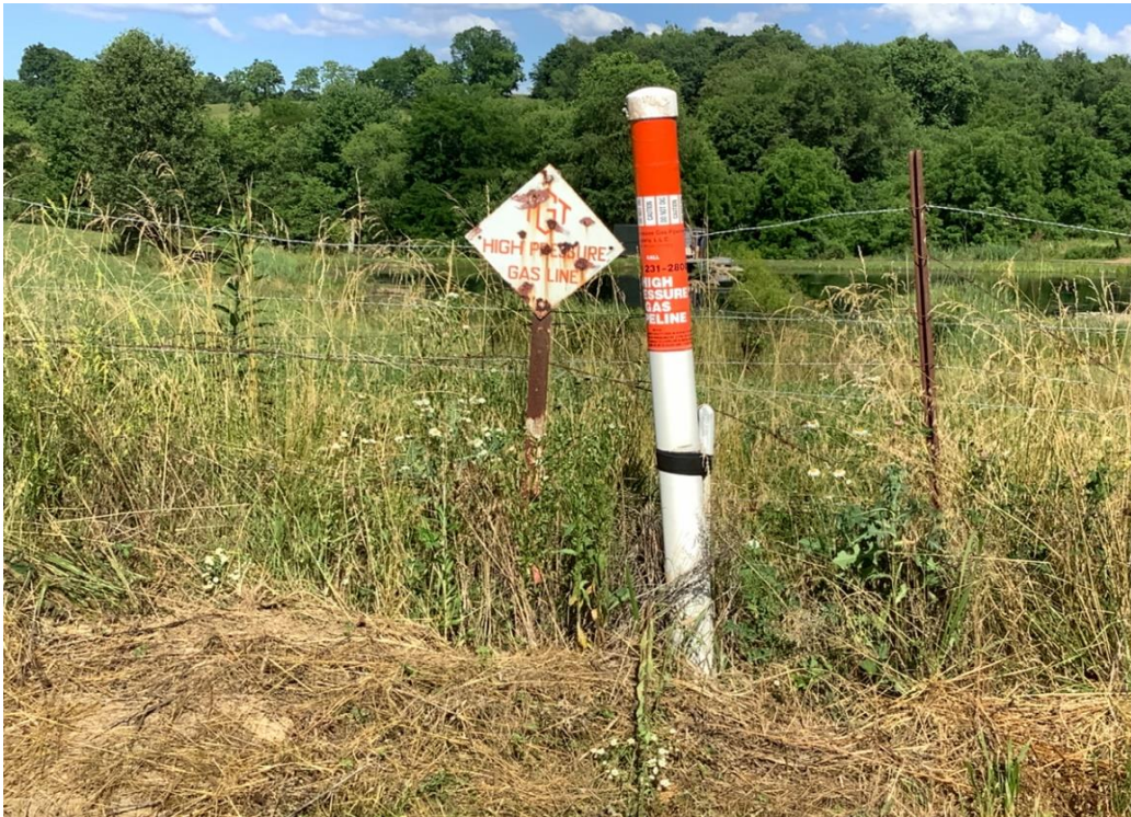
PHOTO 28: Underground high-pressure gas line marker on Luther Jones Road, looking east.
