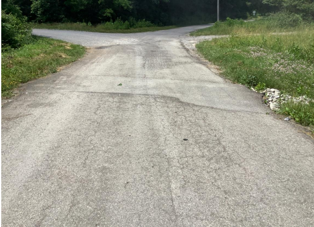
PHOTO 1: Pavement repair over culvert on Dixon Run Road, looking north.
