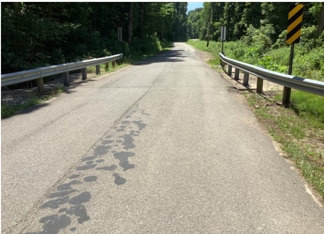
PHOTO 8: View of pavement over Bridge 4034016, looking west.
