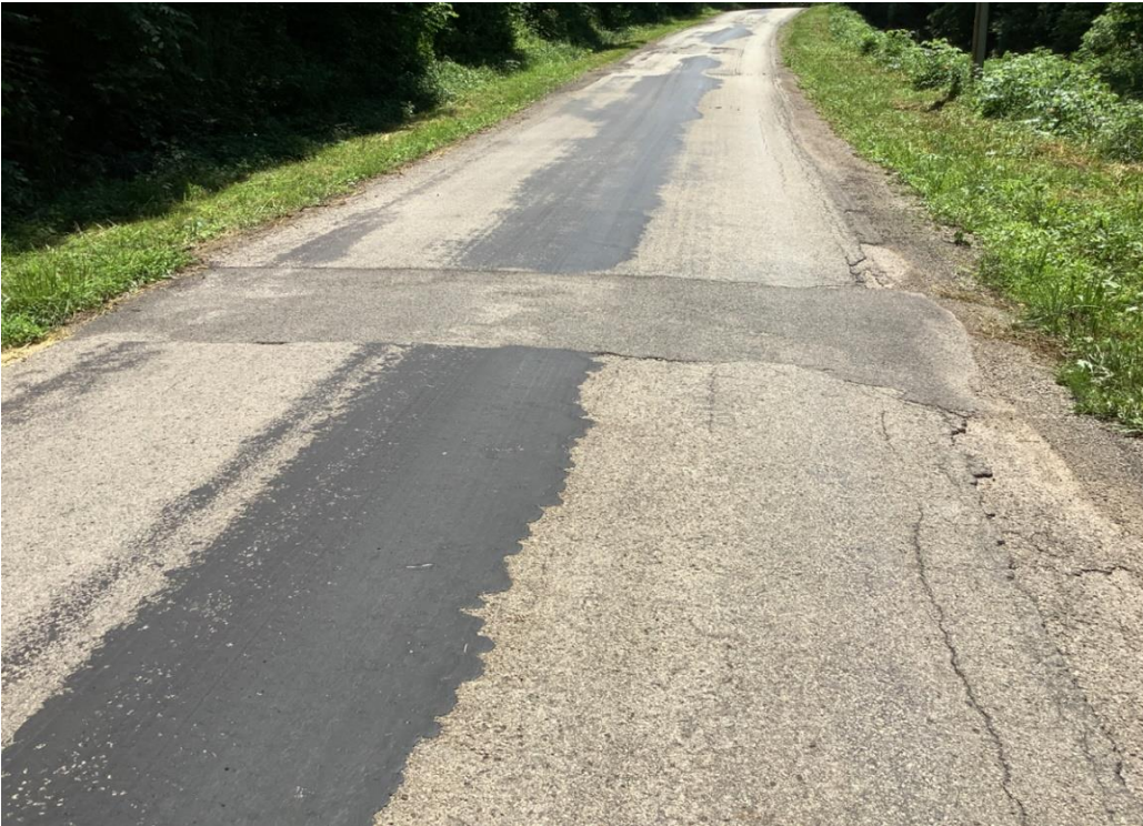
PHOTO 10: Pavement repair over culvert on Dixon Run Road, looking south.
